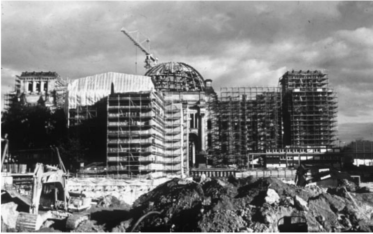
Plate 3.1 The Reichstag during Norman Foster's reconstruction. Photograph: Simon Guy.
