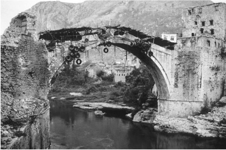
Plate 8.2 The Old Bridge (Stari Most) in Mostar, Bosnia-Herzegovina. The Old Bridge was shelled first by Bosnian-Serb troops and then by Bosnian-Croat troops (who finally destroyed it at around 10.15 a.m. on November 9, 1993). An ultimately unsuccessful attempt was made to protect the damaged bridge by hanging tires around the stonework. Image © Nigel Chandler/Corbis. Used with permission.
