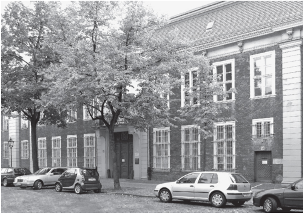
Facade of the Lindenstrasse interrogation prison in Potsdam, now a memorial to all who suffered there. Only the bars on ground floor windows still hint at the suffering that went on there.
